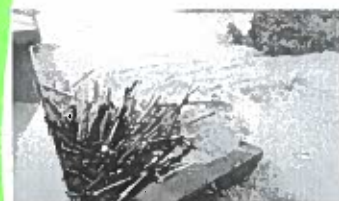
CLOGGED RIVER: A buildup of debris, including plastic trash and bamboo, collects under the Umatac Bridge along Route 2 on Thursday afternoon. A house next to the bridge was flooded with more than 2 feet of water as the nearby river overflowed.
