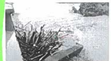
CLOGGED RIVER: A buildup of debris, including plastic trash and bamboo, collects under the Umatac Bridge along Route 2 on Thursday afternoon. A house next to the bridge was flooded with more than 2 feet of water as the nearby river overflowed.
